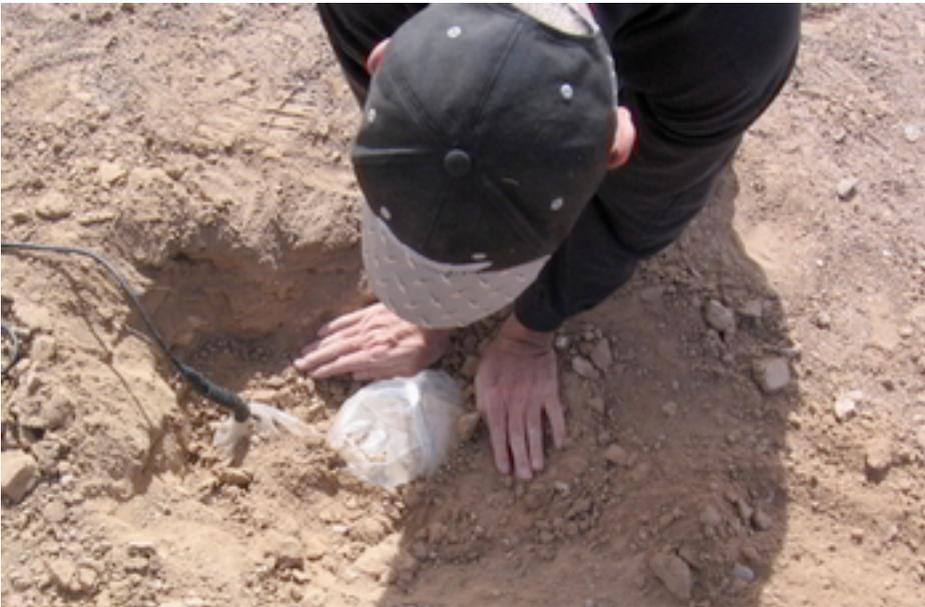
Carefully fill in the rest of the dirt around and over the L-22 using your hands.
