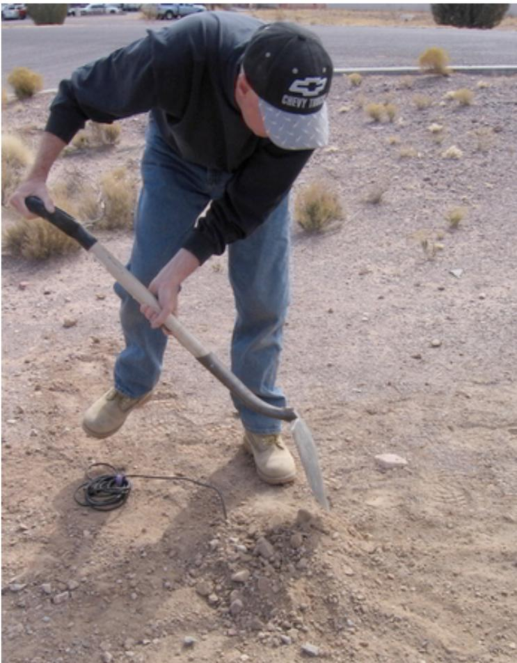
Mound more dirt over the sensor pit to help drainage away from the sensor. Dig a small trench from the sensor to the digitizer for the sensor cable. Beware! Do not cut the sensor cable with the shovel. Carefully bury the sensor cable to guard against wind noise and animals.
