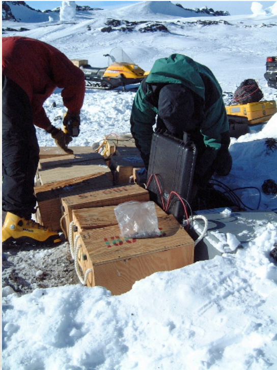
Batteries at the Truncated Cones seismic station. (Photograph Courtesy of Jessie Crain - 2001)
